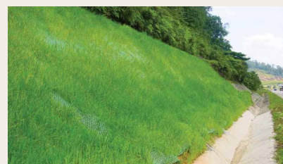
A vegetated reinforced soil slope with Polyfelt® Polymat EM.
