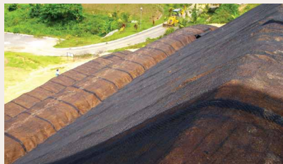
TenCate Polyfelt® Envirofelt laid over a reinforced soil slope.
