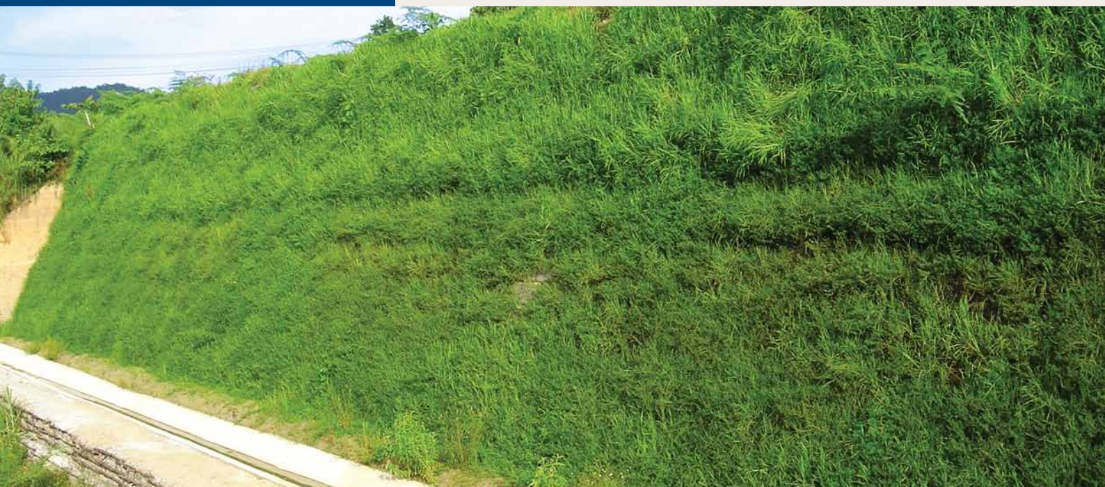
A vegetated reinforced soil slope with Polyfelt® Polymat EM.
