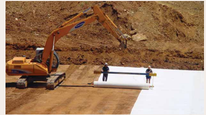
Laying Polyfelt® Enviromat GCL using crane.
