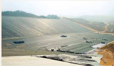
Installing Mirafi® FW across a major landfill.
